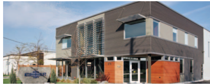
PHOTO CREDIT: GORDON KING/CHRISTOPHER SIMMONDS ARCHITECT INC.
