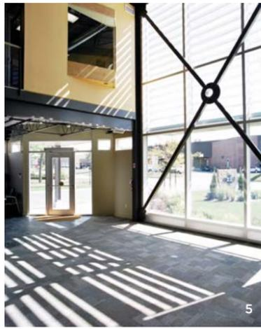
LIGHT STREAMING THROUGH THE LARGE SOUTH WINDOW, BRACED FOR LATERAL RIGIDITY, REDUCES HEATING REQUIREMENTS AND CREATES A VIBRANT INDOOR ENVIRONMENT [5]. THE VIEW OPPOSITE PHOTO 5, NOTE HOW THE INTERIOR OFFICE WINDOW ANGLES TO CATCH THE NATURAL LIGHT [6].
